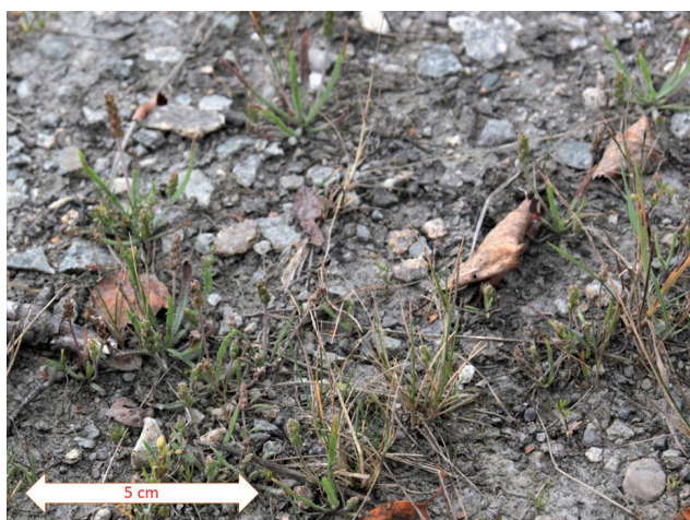
Fig. 7 Tiny plants of Plantago coronopus and Puccinellia distans created a sparse vegetation in the plot covered with recycled gravel and old crushed asphalt.
